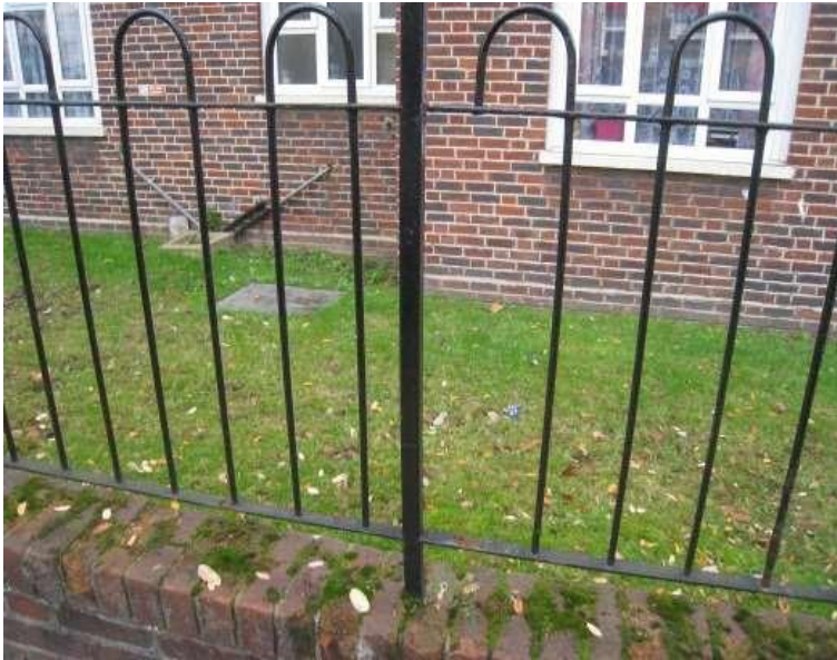
Above: Dwarf boundary brick wall requiring repointing and cleaning off of moss growth. Hairpin railings requiring repairs and redecoration
